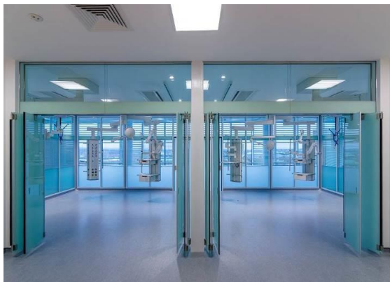
Picture 3: Central work stations of the new CCU
